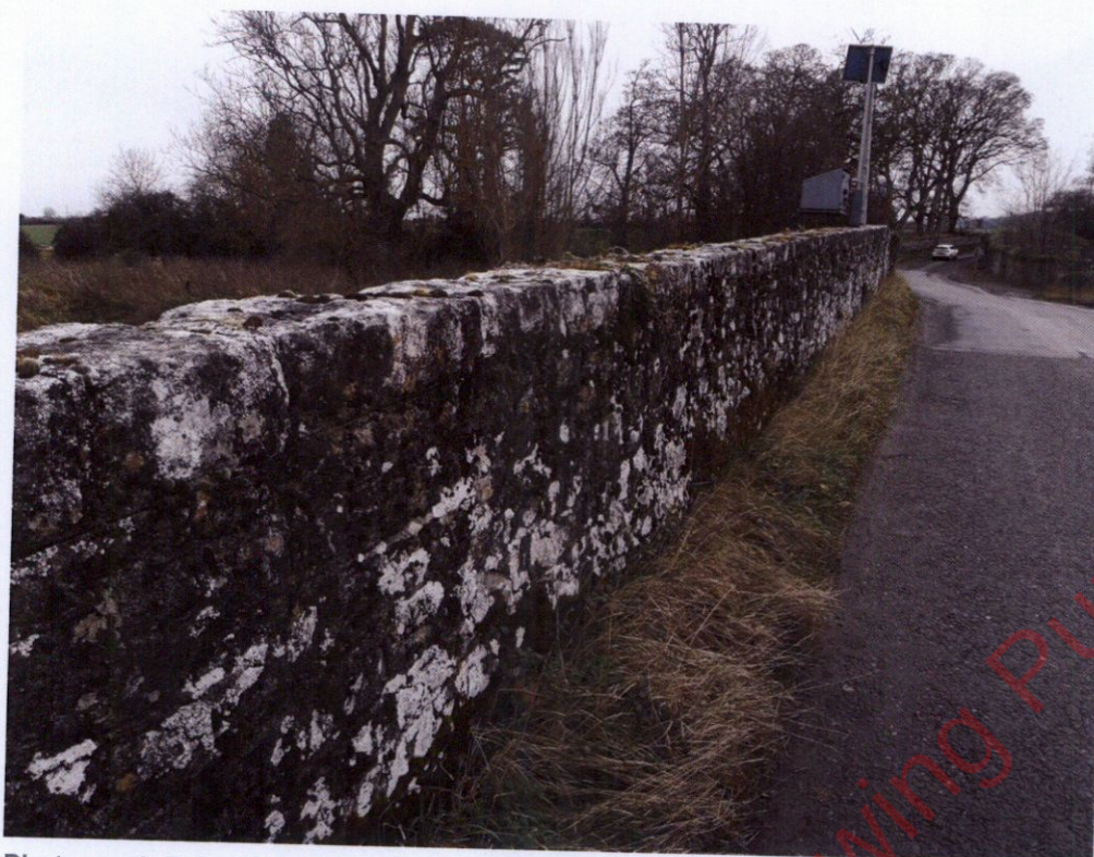
Photograph B-5 – East parapet and grass verge
