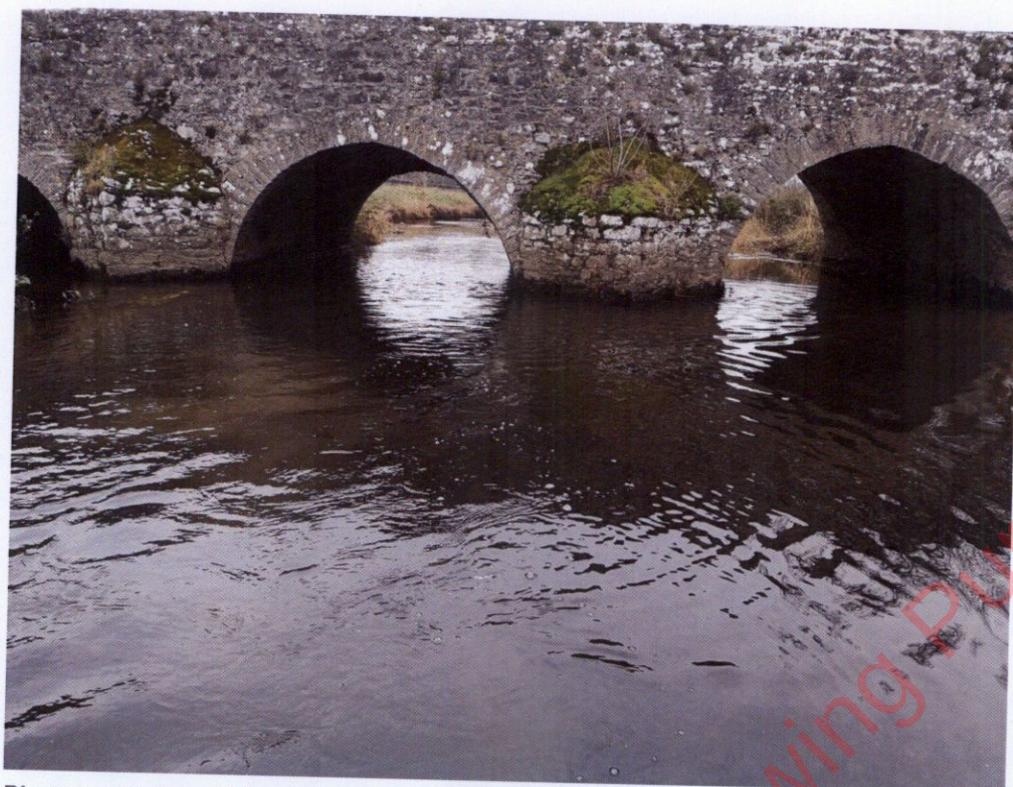
Photograph B-31 – View of upstream riverbed with watercourse main channel through arches 3 and 4
