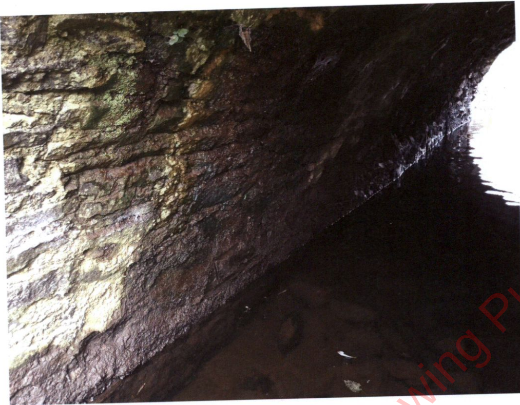
Photograph B-21 – South face of pier 5
