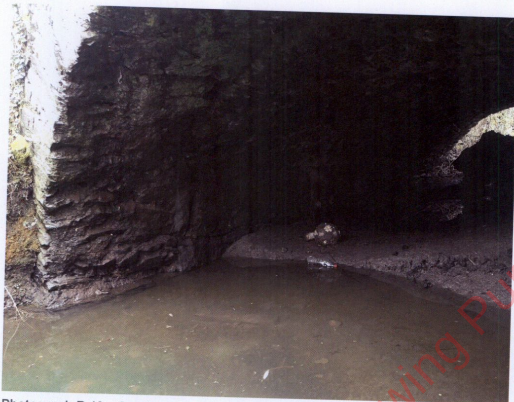
Photograph B-13 – South abutment
