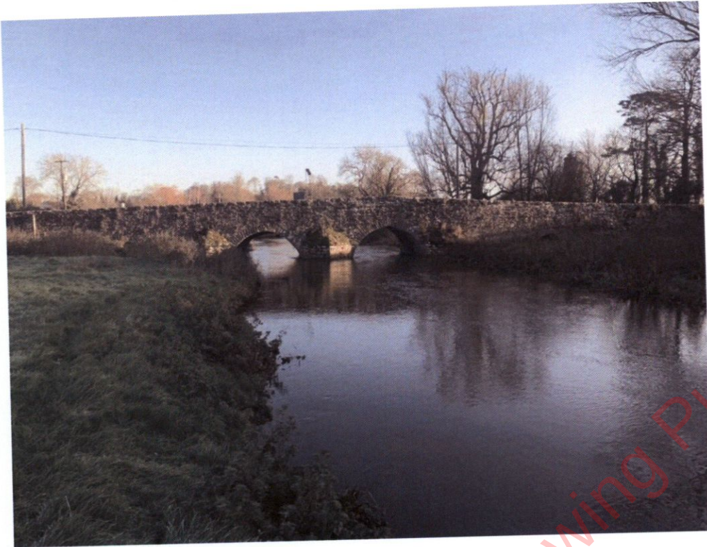
Photograph B-33 – View of west elevation
