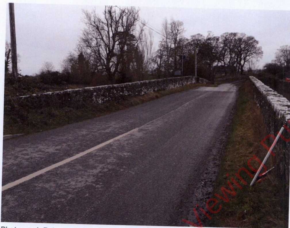
Photograph B-1 – Bridge surface looking south
