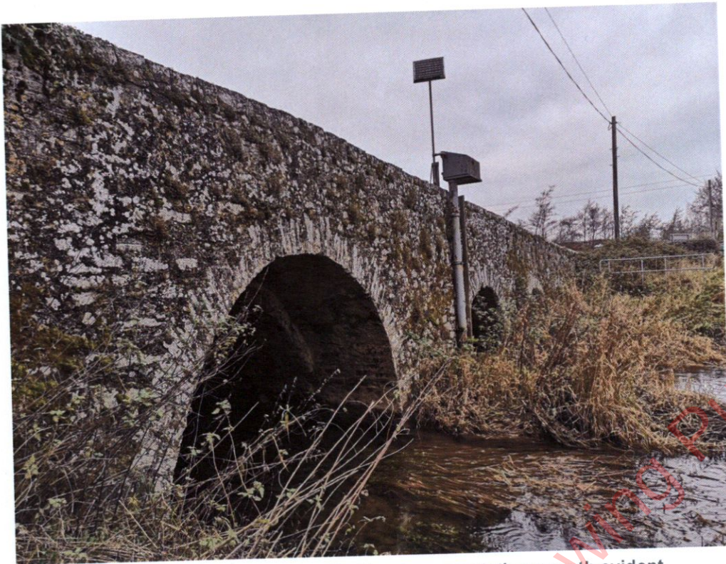
Photograph B-11 – East spandrel wall with minor vegetation growth evident
