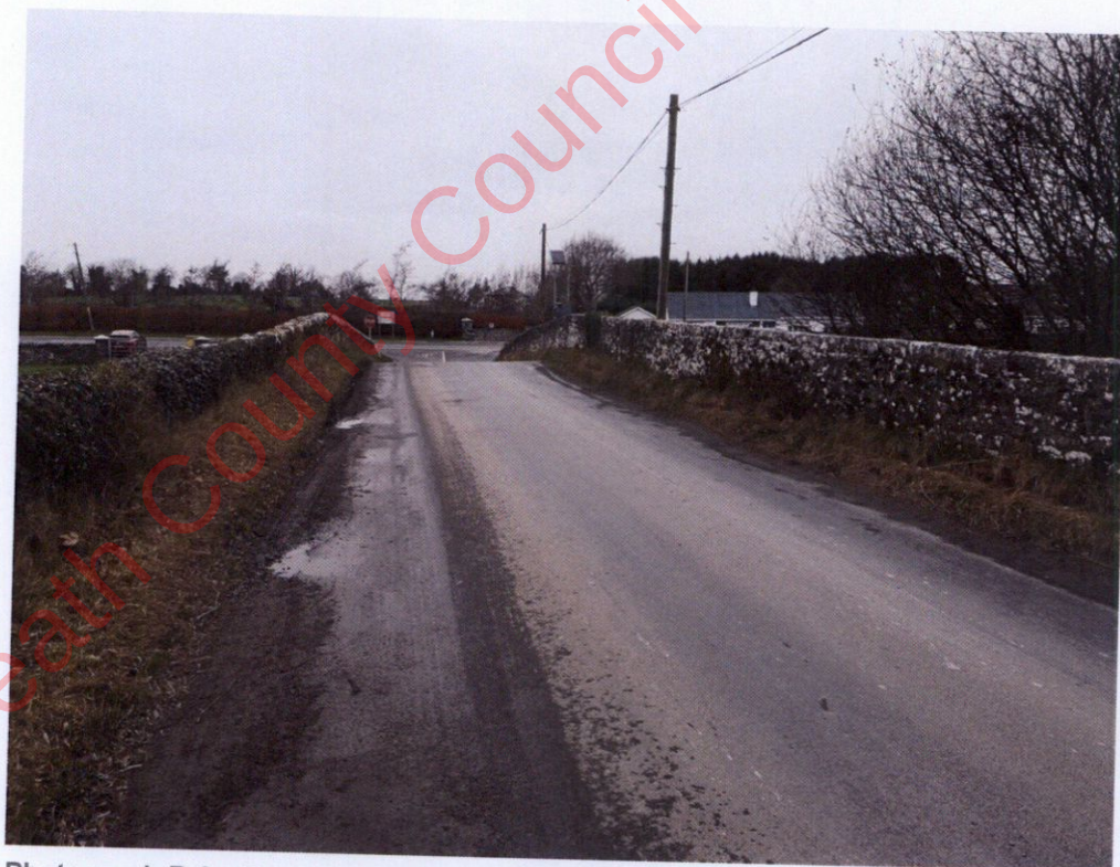
Photograph B-2 – Bridge surface looking north
