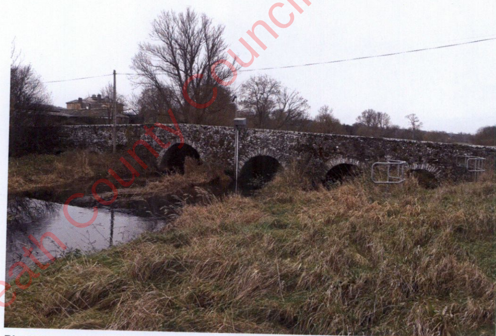
Photograph B-32 – View of east elevation
